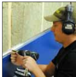
7 Mounting a connecting profile.
