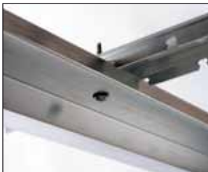
5 Secure snap lock with selfdrilling
