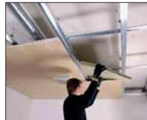
7 *Install mineral wool insulation.
