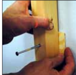
2 Adjust the battens with the help of spacers.
