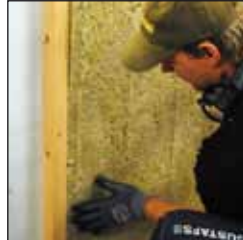
3 *Installing the insulation.
