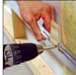
4 Setting out the first Capax onto battens.
