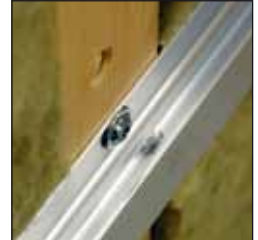
5 Remove any dust or filings from the Capax.
