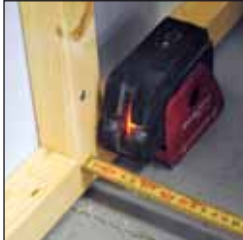
1 Mount the battens with the help of a laser.
