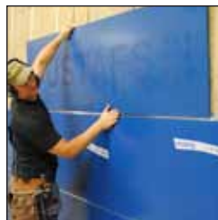
8 Installing the next panel.
